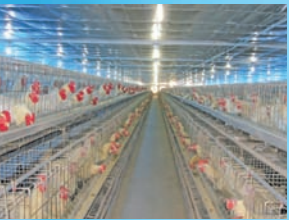
Poultry House Project
